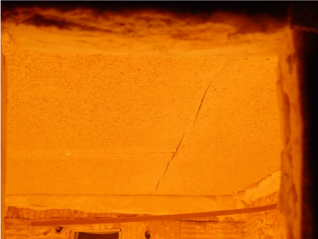
65 minutes: E-W joint at N end of furnace
