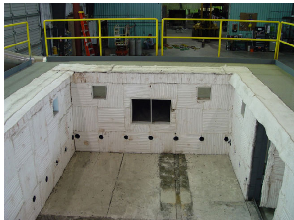
Figure 2: Large-Scale Horizontal Furnace Interior View
