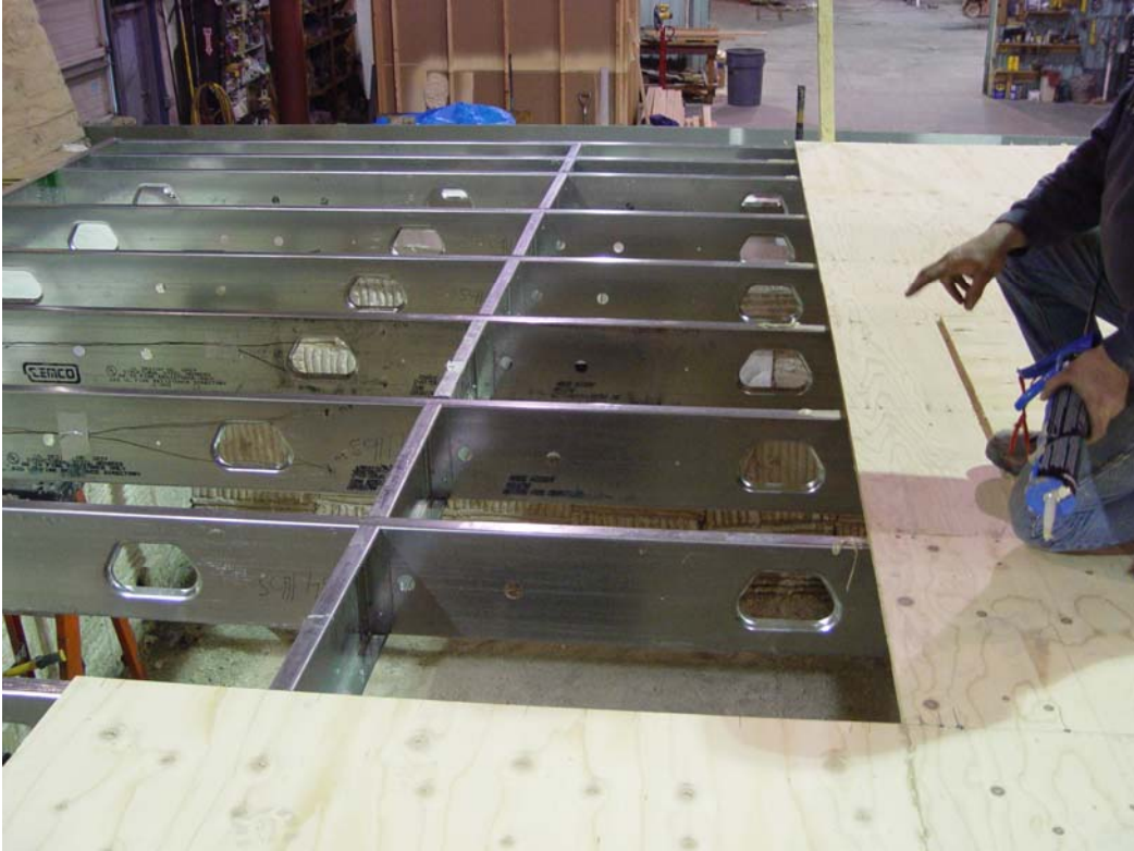
Placement of Subflooring Atop Steel Joists
