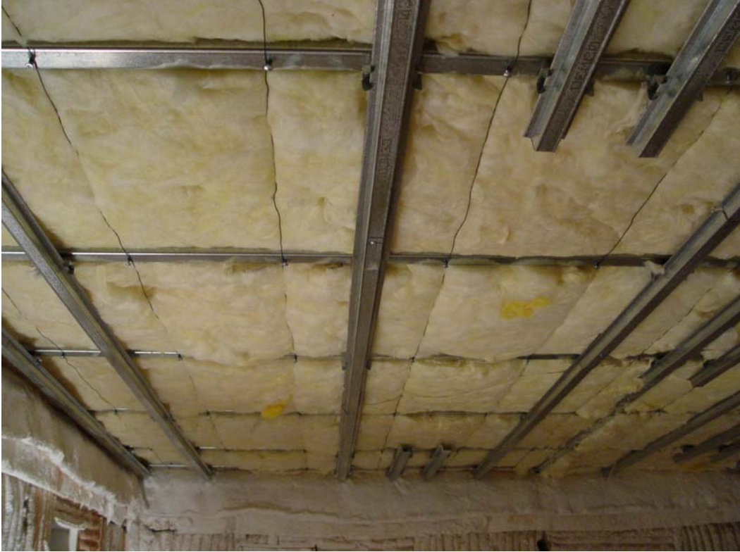
Insulation and Furring Channel Placement
