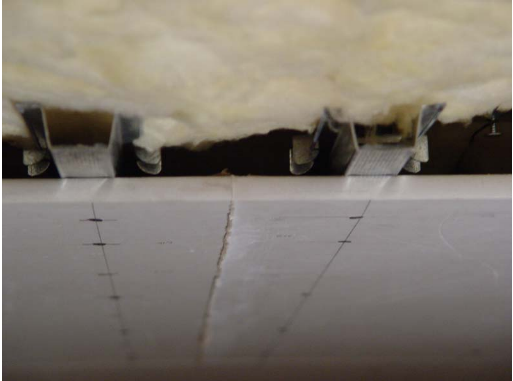
Base (Upper) Layer Butt Joint
