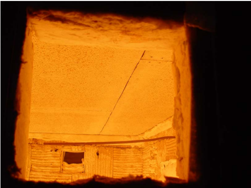
30 minutes: E-W joint at N end of furnace
