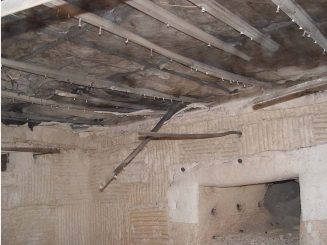
NW qtr section with furring channel and insulation exposed
