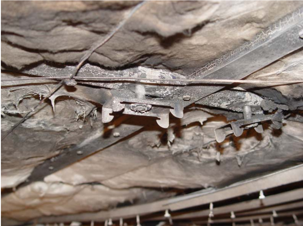
RSIC-1 clips with channel removed
