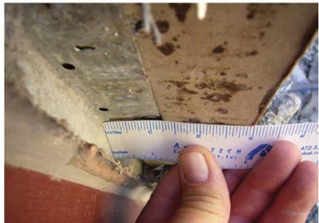
Water can enter through the perforated nail holes on the casing bead.
