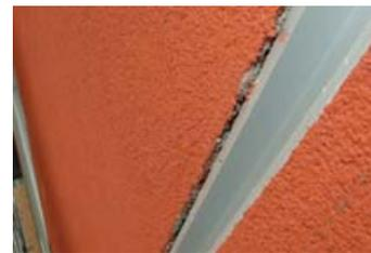
Cement stucco pulling from aluminum leaving large enough gaps for bulk water to enter the stucco.
